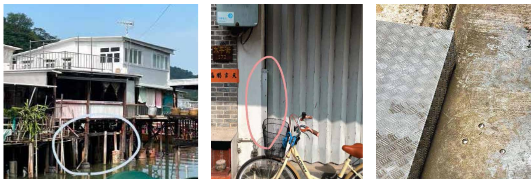
(Left) Gaps between poles that hold up stilt houses (taken by the research team) (Middle) Water gates at the doorway (taken by the research team) (Right) Screws on the ground for temporary barriers to be inserted (taken by the research team)
