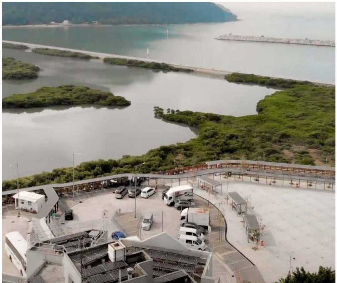
Elevation of Car Park (taken by res Aerial Shot of Lung Tin (taken by research team))
